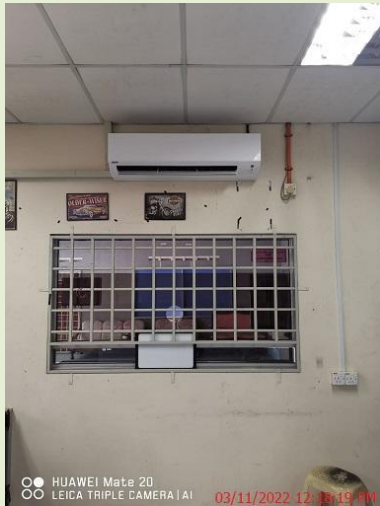
Pemasangan unit wall mounted di C4
